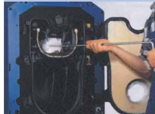
The full swing burner door on the combustion chamber allows for easy, thorough and proper cleaning in a fraction of the time it takes to clean a conventional boiler.
